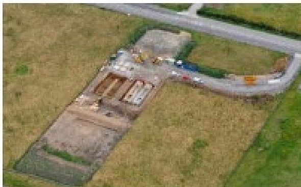
EXAMPLE OF TRANSITION JOINT BAY UNDER CONSTRUCTION
