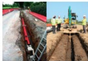
Image left: Typical 110kV Trench Excavation (Ducts in Trench Formation).
