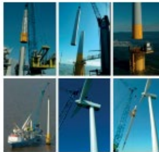
Sequential photographs of installation of turbine tower, nacelle and blades.
